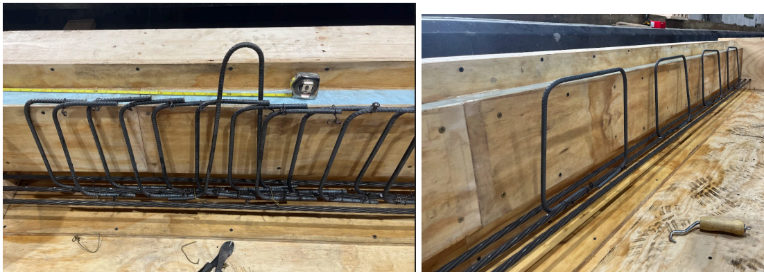
Figure 6: Shear Reinforcement
